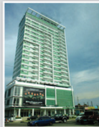
INJAP Tower Hotel by DoubleDragon Properties Corp.
