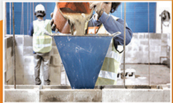
Every 3-4 rows, flowable concrete grout is poured into the block cavities. A Smart Wall then becomes reinforced and load bearing.
