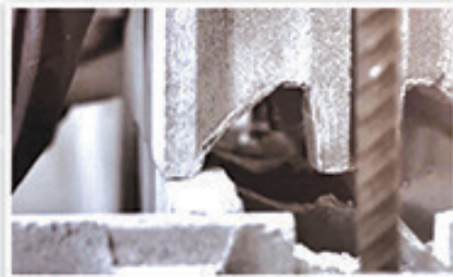
Grooves on the top and bottom of the blocks ensure precise horizontal alignment.
